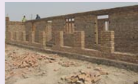
A Hidaya school under construction - July, 2007
